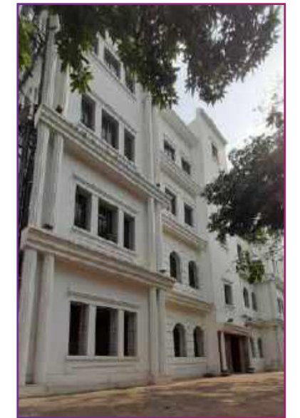
Lord Sinha Road Office – Certified as LEED v4.1 Gold in 2023 by USGBC
